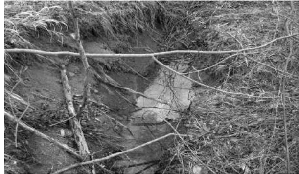
Fig. 9. Pond formed in a transverse crack
