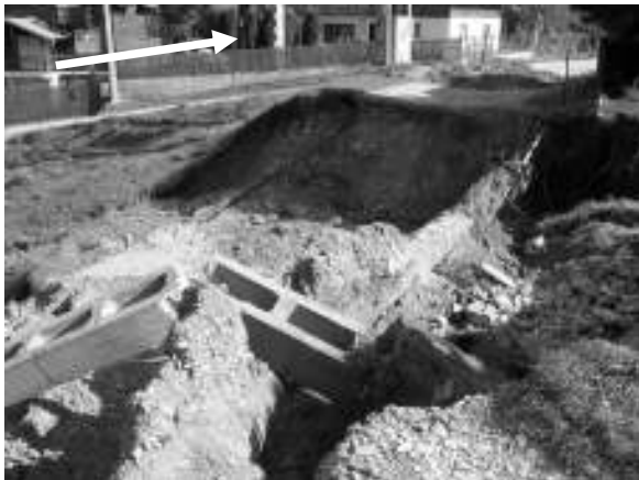
Photo 2 The landslide at the margin of the Alecsandri Street (September 2005); the paths of the pipes and electric cables that led to slope instability; in the right side, the cobbles of a well felt into the breaking crevice
